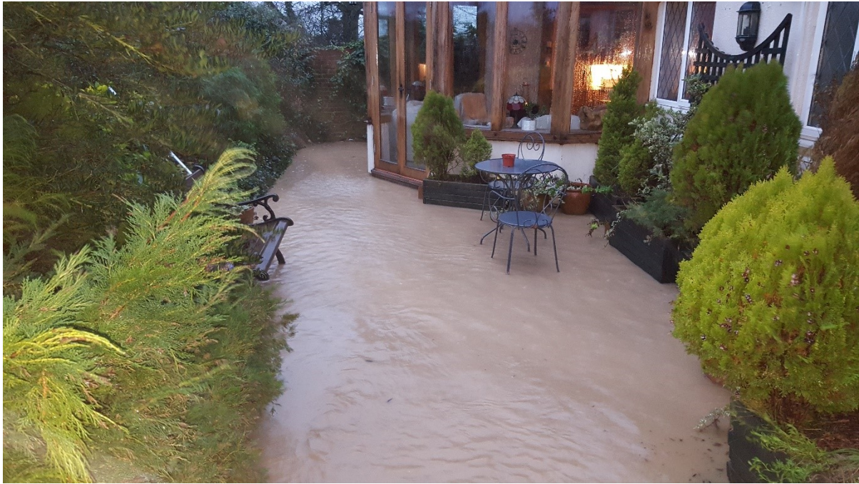
Figure 2 Flooding at Bow Cottage
